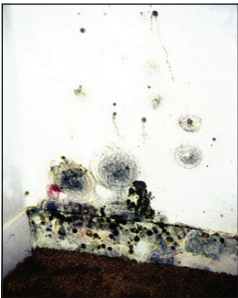
Mold damage.
