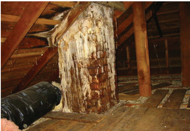
The most important step in solving a mold problem is to identify and correct the moisture sources that allowed the growth in the first place.
